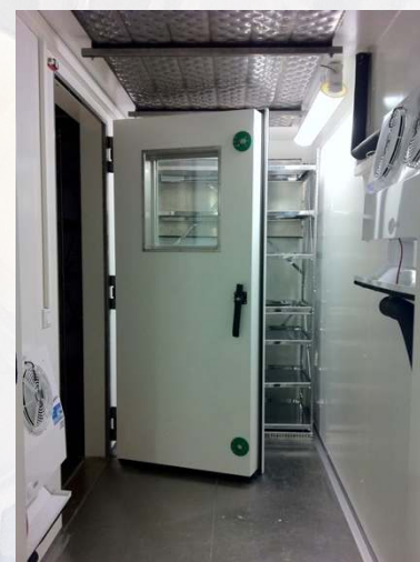
View from the load lock chamber (-20°C) into the storage room (-80°C)
